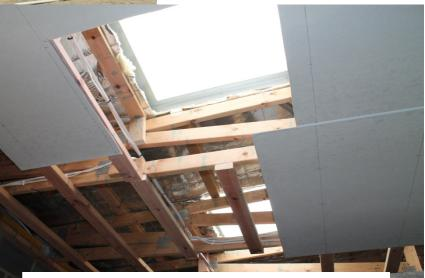
The skylights are being installed and the lining of the ceiling has commenced.
